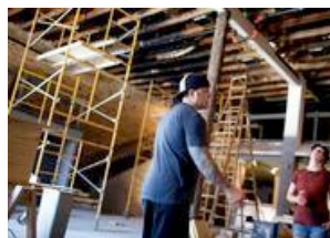
A Look Inside Renovations At Trees
